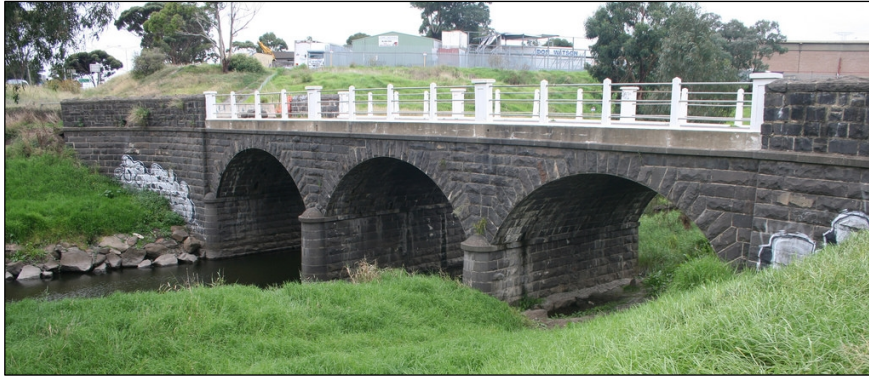
Figure 1 Melbourne's Brooklyn Bluestone Bridge (Source: williewonker Flickr 5612800971_84840674bd_b)
