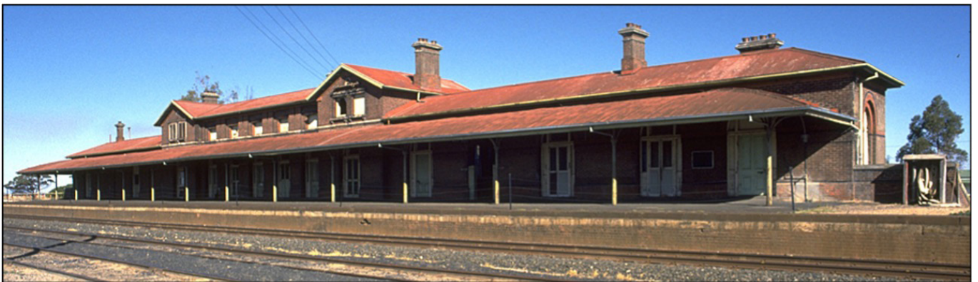
Serviceton station (Source: www.kaniva.org/serviceton-station.html )
